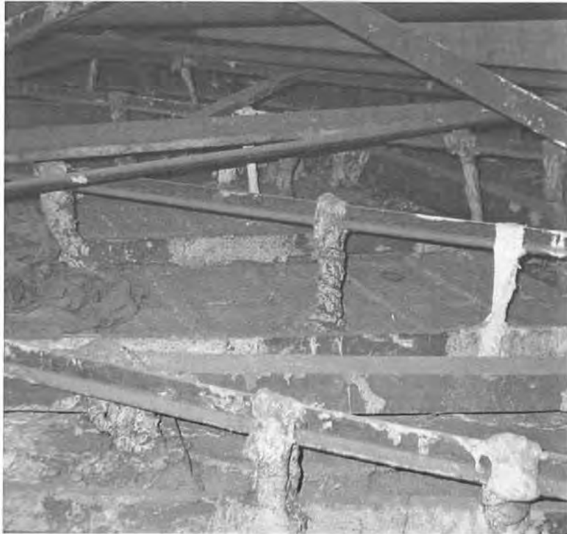
Plate 24 Typical wadding tie suspension system using hessian soaked in plaster of Paris. Photo courtesy of English Heritage in Mortars Renders & Plasters (2012) p.109
