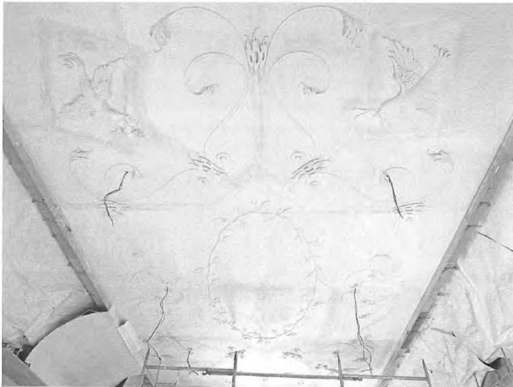
Plate 20 Suspension and making good of modern 24 panel fibrous plaster ceiling bed 2012
