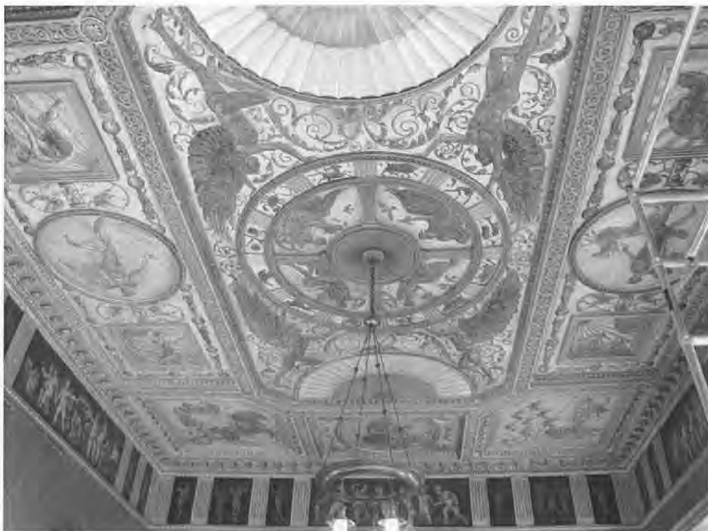
Plate 23 Walter Crane ceiling installation at Combe Bank Sevenoaks
