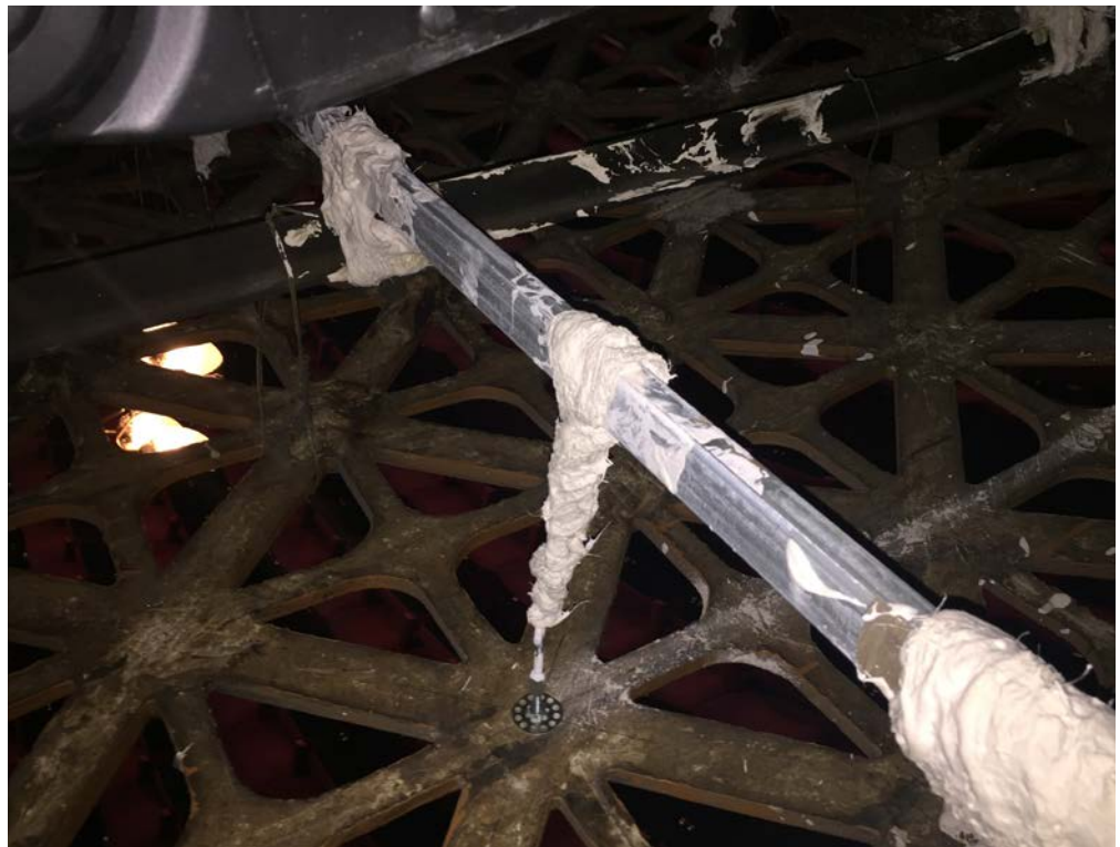
Figure 33: Fibrous plaster fretwork, given supplementary support with a new beam and wire-reinforced wads. This is a standard method of improving the stability of suspended ceilings.
