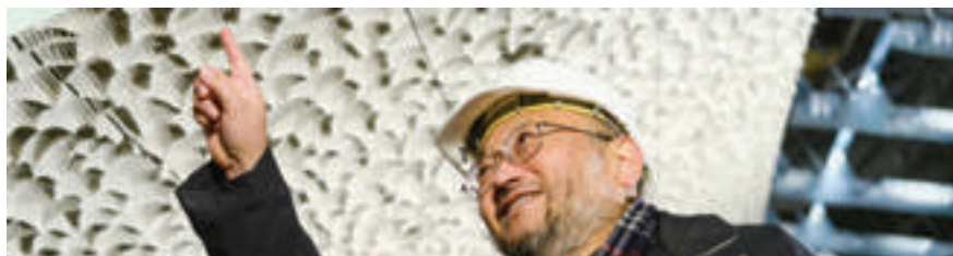
Micro-shaping surface diffusion is an effect above 9kHz and is inaudible
