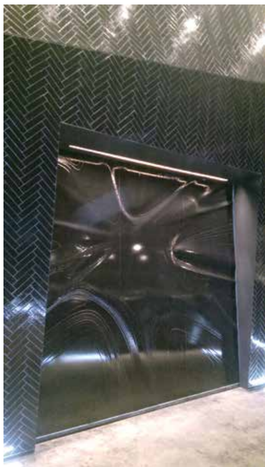
Fire rated acoustic sliding door, National Sawdust, NY
