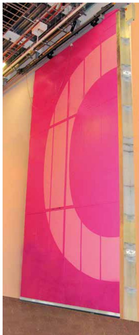
Liverpool Everyman Pivot door in hold open position in corridor (far left) Wales Millenium Single Horizontal Sliding Rw56dB 1 hr Fire Door (left)
